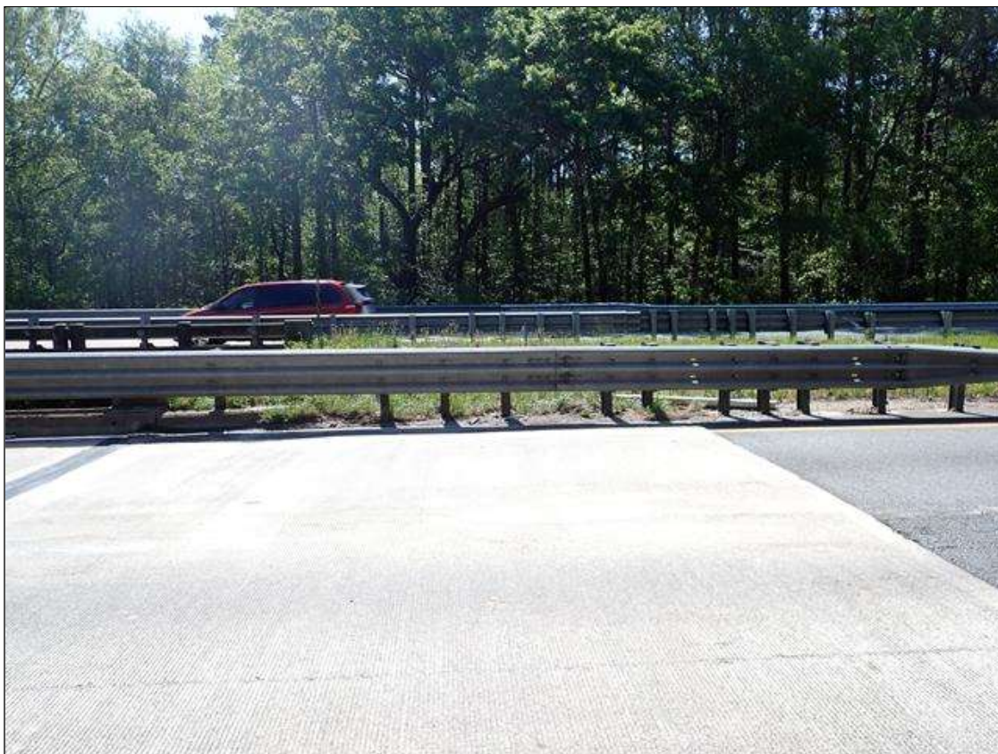
South East Guardrail Transition, Typ.
