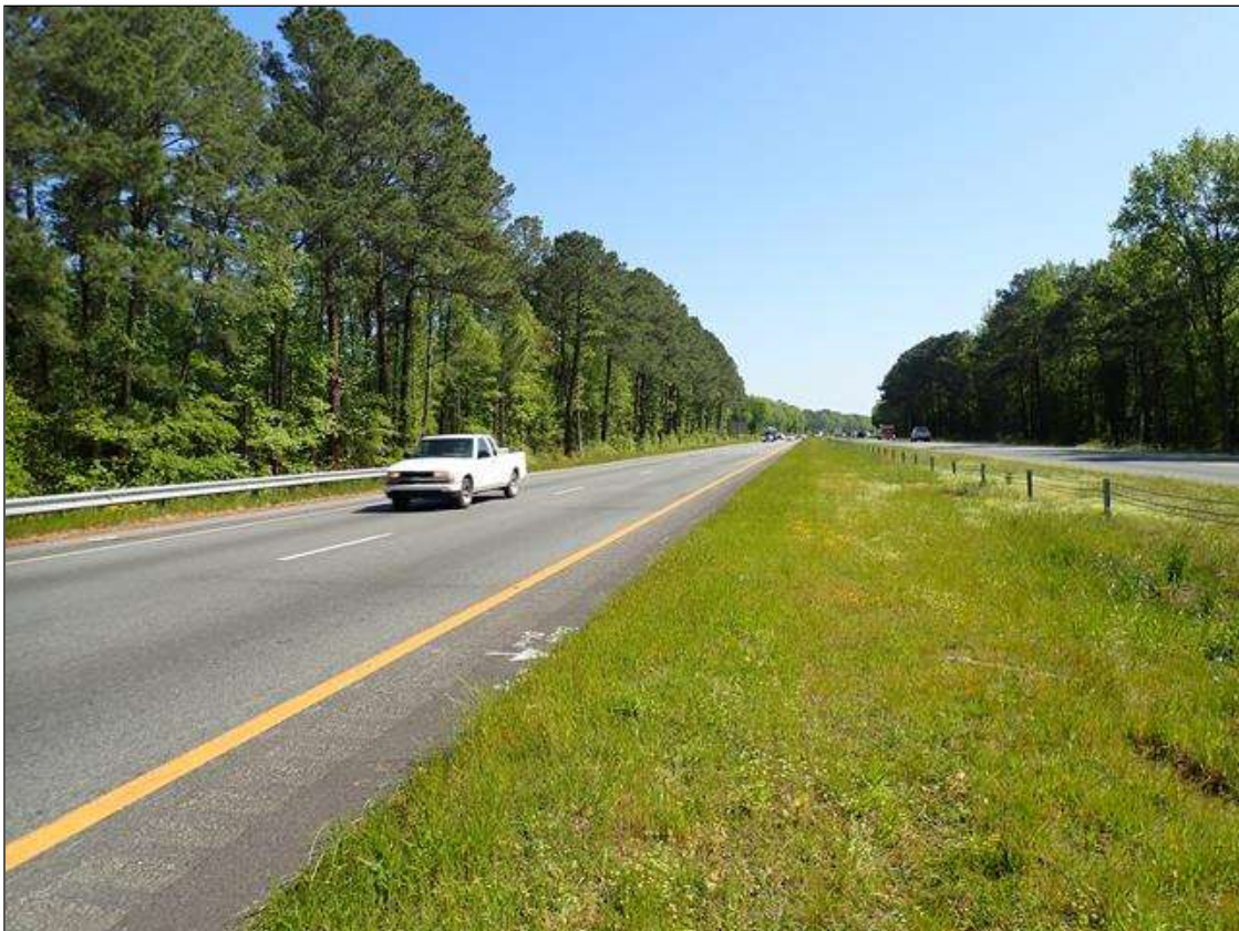
North Approach looking North
