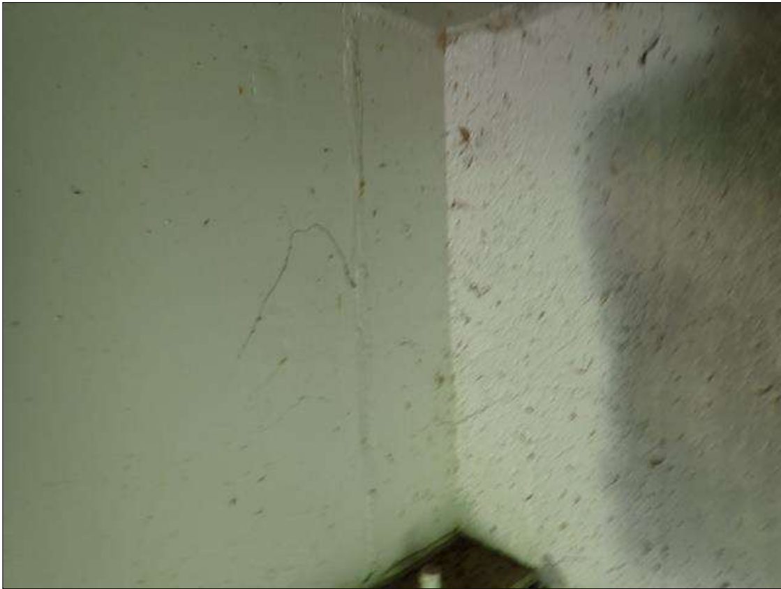
Span 1 Beam 2: 7" x 31" area of replaced beam at End Bent 1
