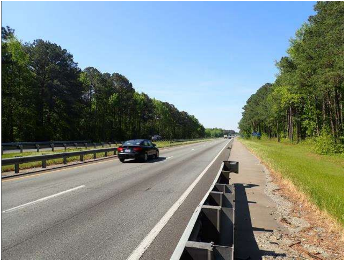
South Approach looking South
