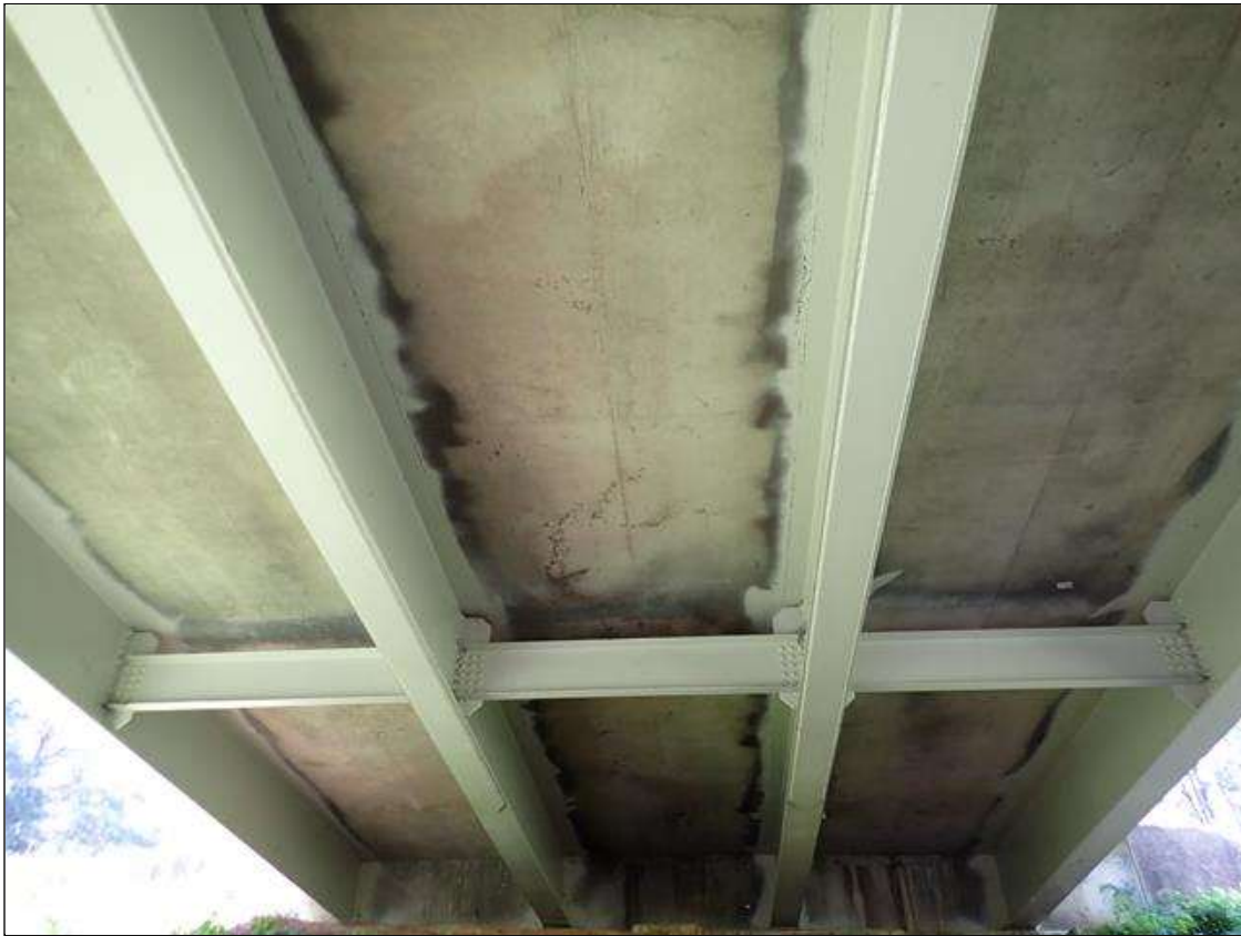
Underside of Superstructure Span 1 (Typical)
