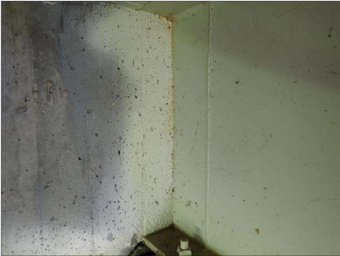
Span 1 Beam 1: 7" x 31" area of replaced beam at End Bent 1
