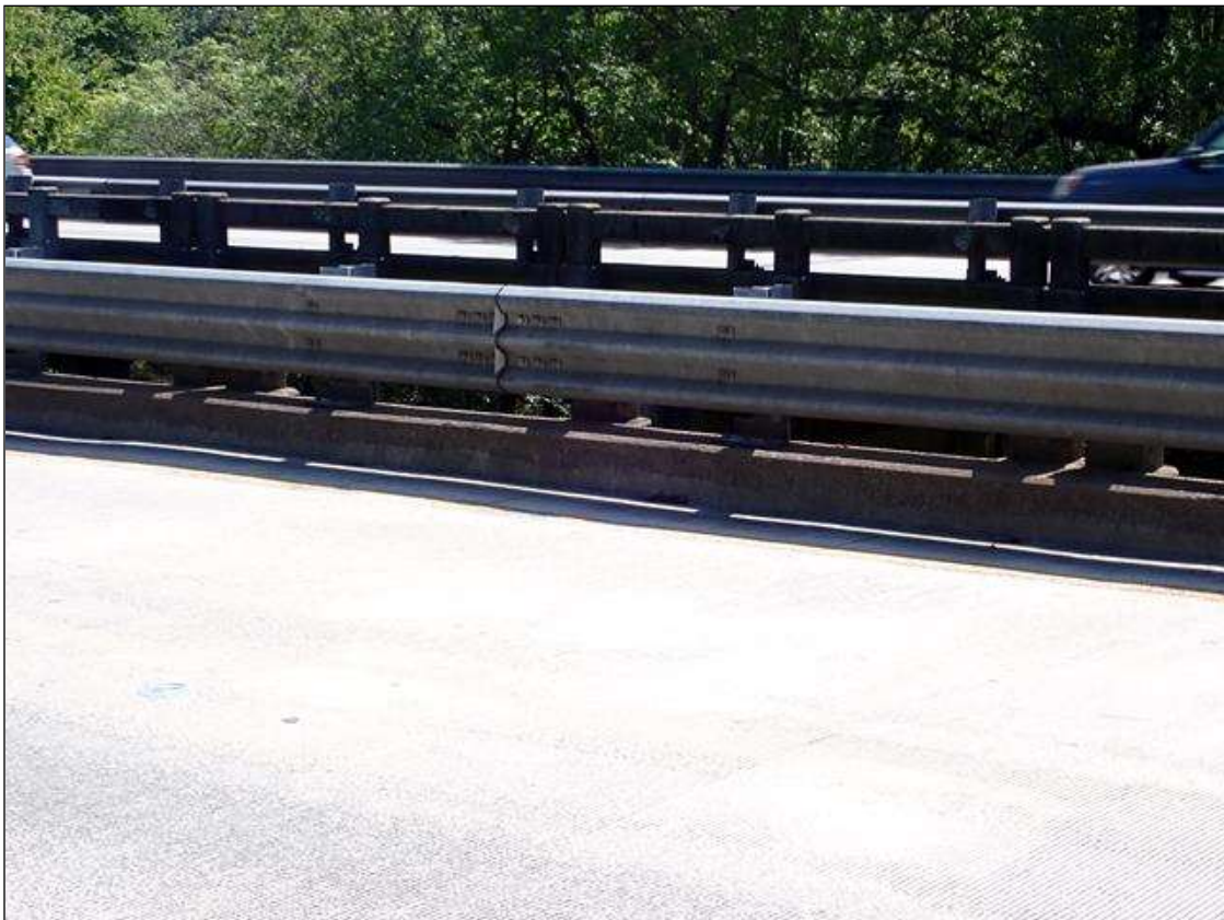
Right Barrier Rail
