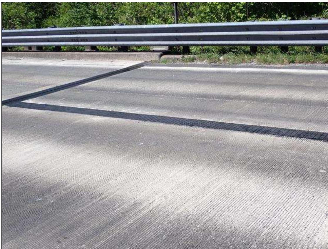
Approach 2 : REPAIR MADE TO CRACK IN CENTERLINE OF APPROACH SLAB
