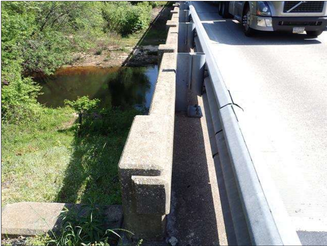
South West Guardrail Attachment, Typ.
