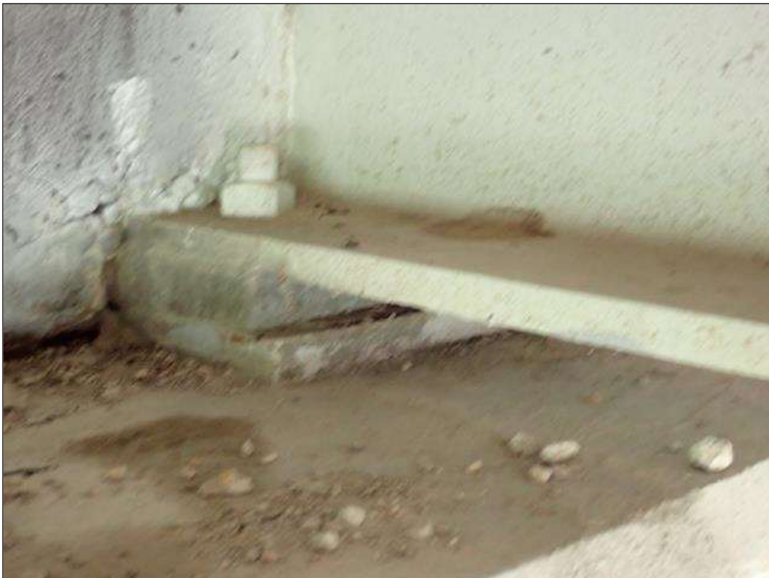
Typical End Bent Bearing, End Bent 2
