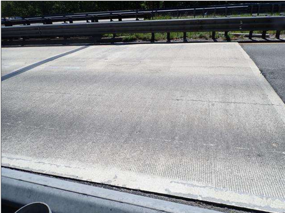
South Approach Slab
