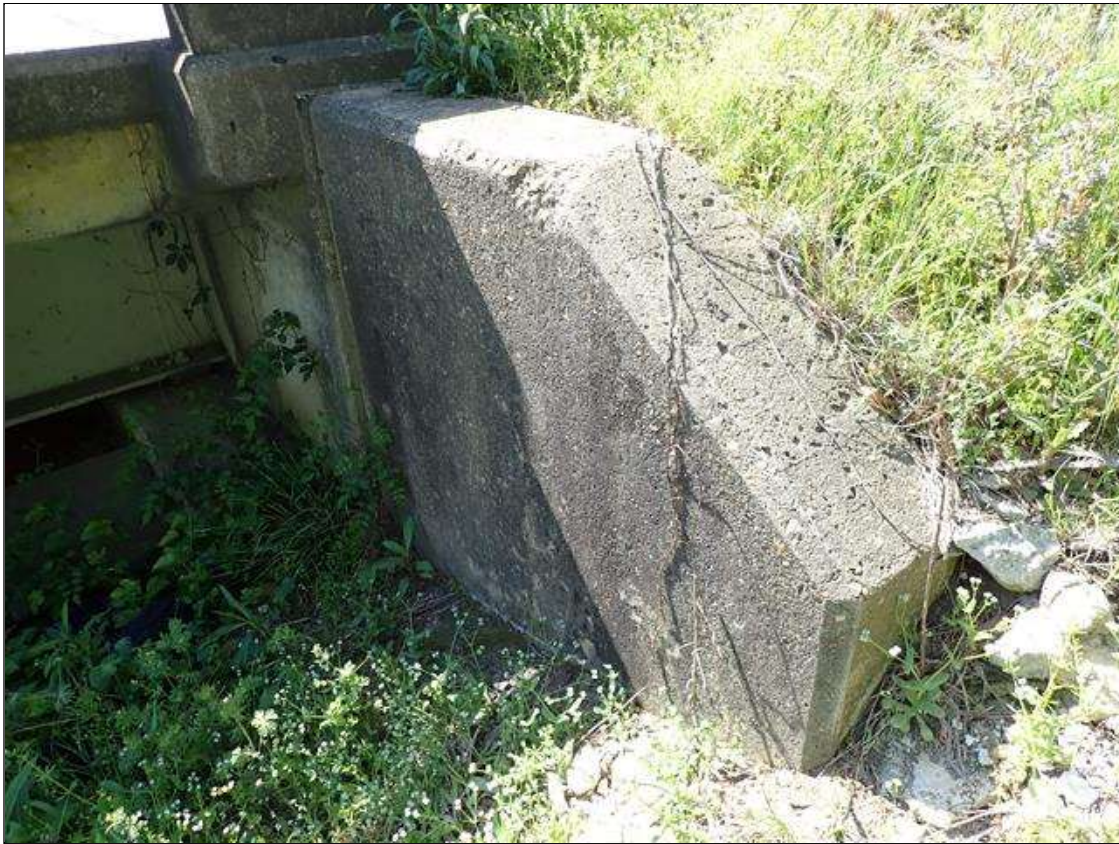
South West Wingwall, Typ.
