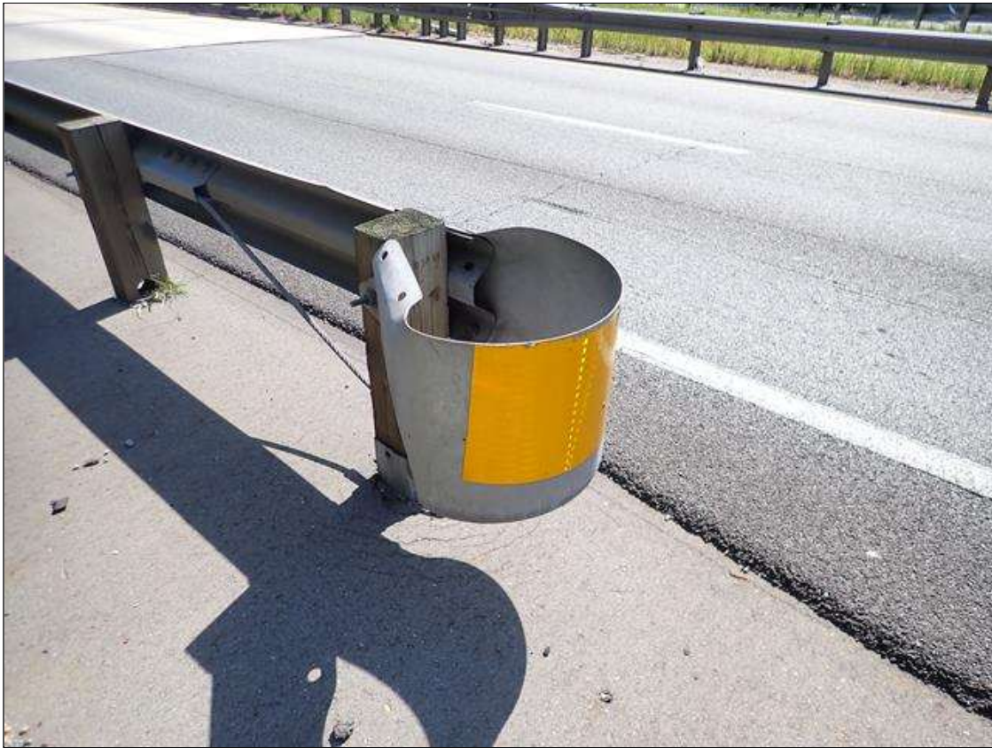
South West Corner Guardrail Termination (South East Similar)
