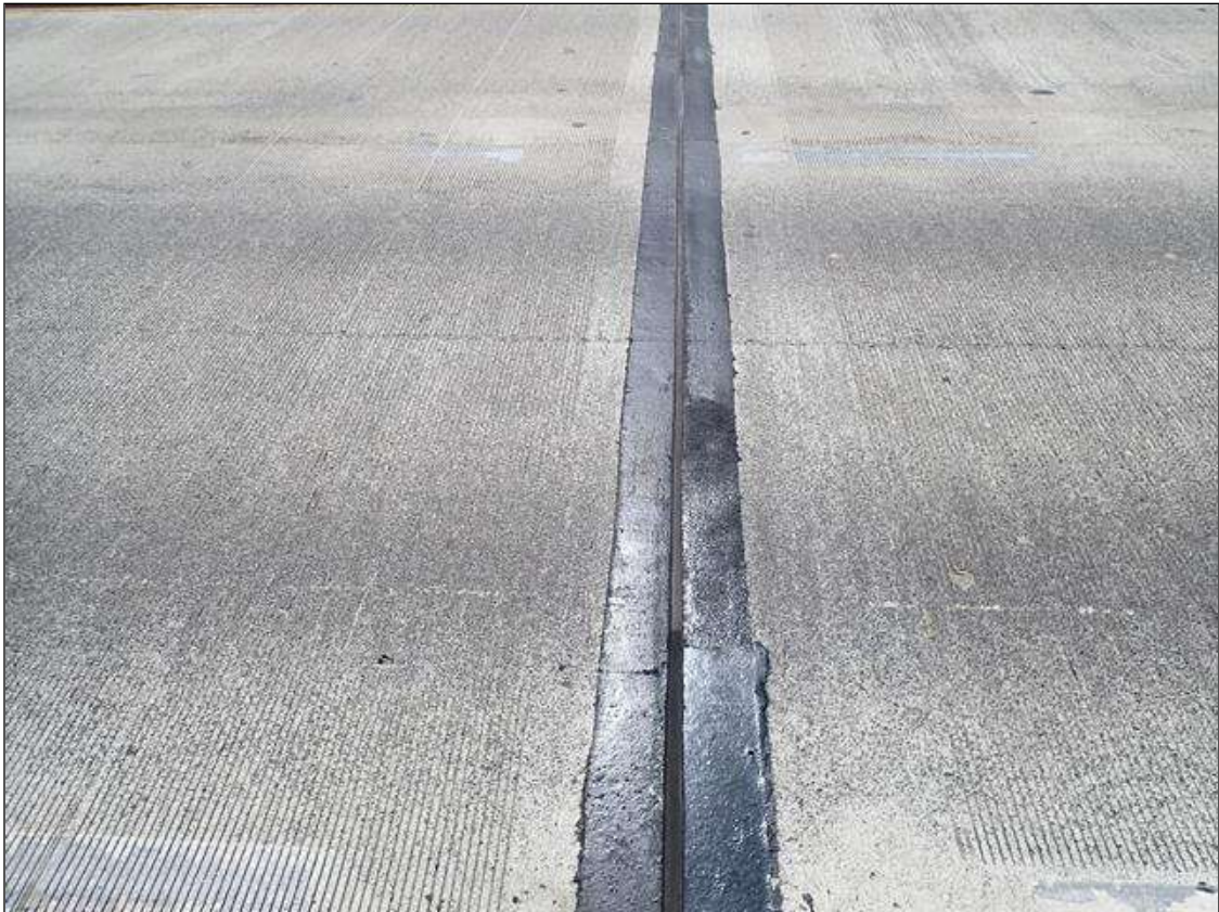
Joint at End Bent 1 (Bent 2 Similar)
