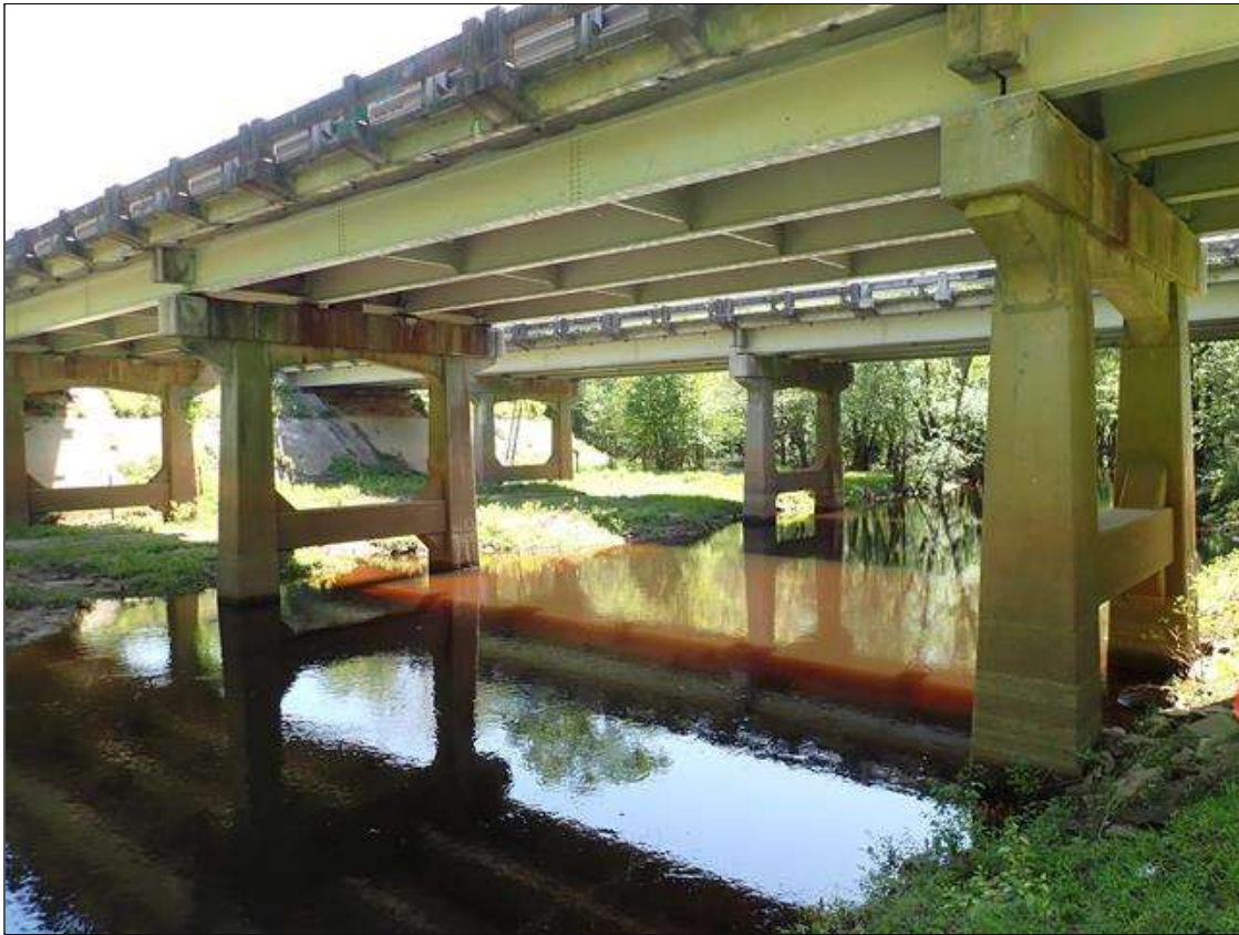
Water Way Opening Upstream looking thru Span 2
