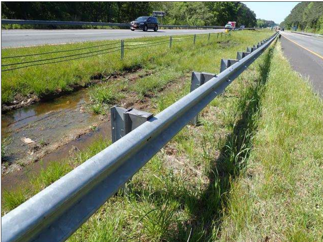
North East Guardrail Post Spacing, Typ.
