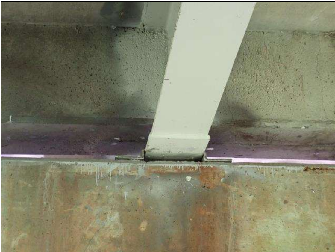
Span 1 Beam 2: 20" x 12" X 3/8" plate welded to bottom flange at Bent 1
