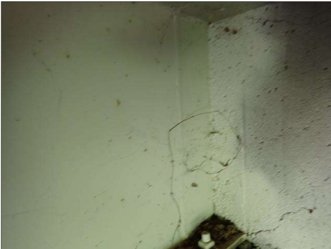
Span 1 Beam 3: 7" x 31" area of replaced beam at End Bent 1
