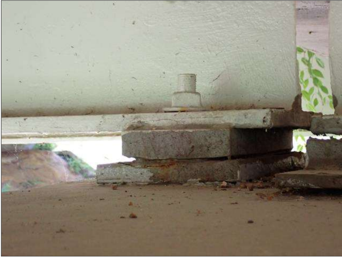
Typical Bent Bearing
