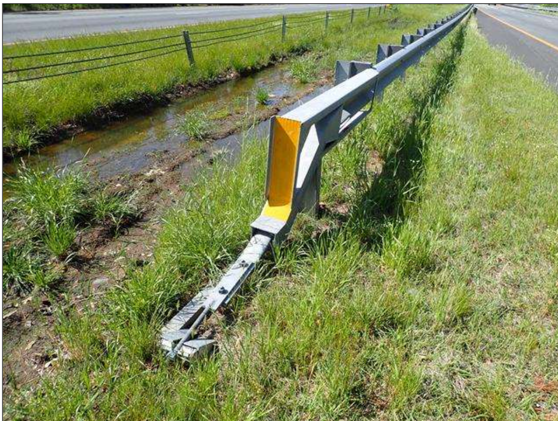
North East Corner Guardrail Termination (North West Similar)
